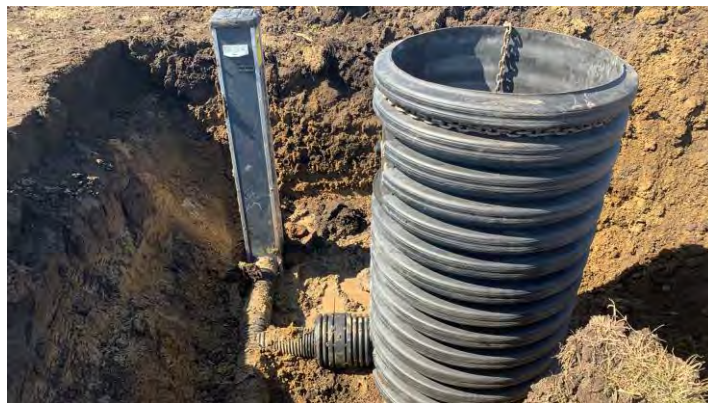
Figure 3. Gate Structures to Control Water Table
