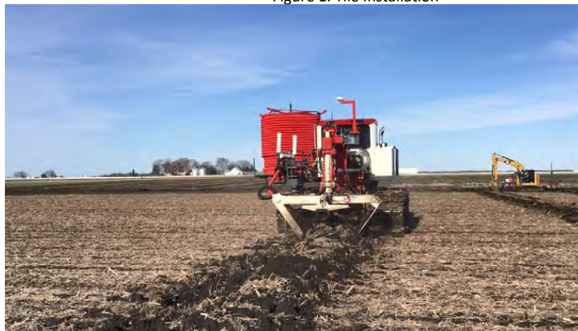
Figure 1. Tile Installation
