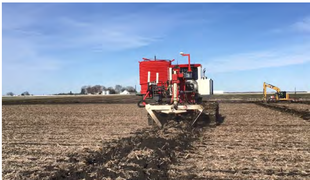
Figure 2. 15' and 30' Pattern Tile Installation
