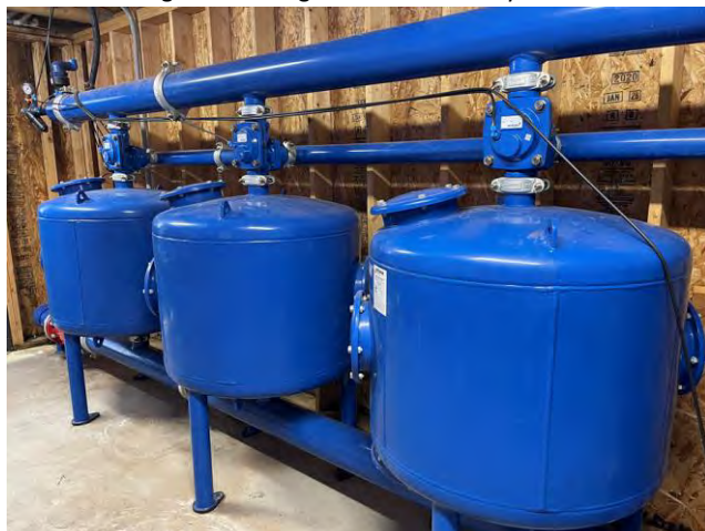
Figure 9. 3-Stage Sand Filtration System
