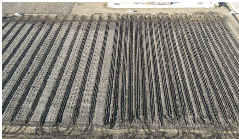
Figure 2. 15' and 30' Pattern Tile Installation
