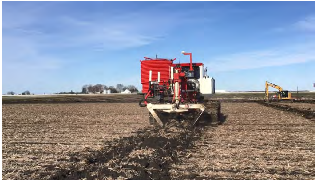
Figure 2. 15' and 30' Pattern Tile Installation
