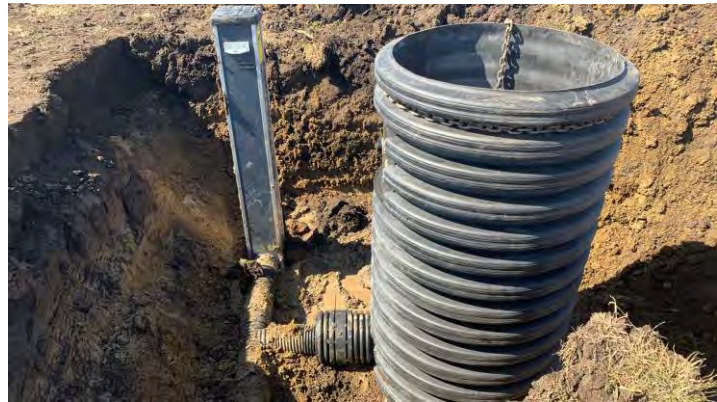
Figure 3. Gate Structures to Control Water Table
