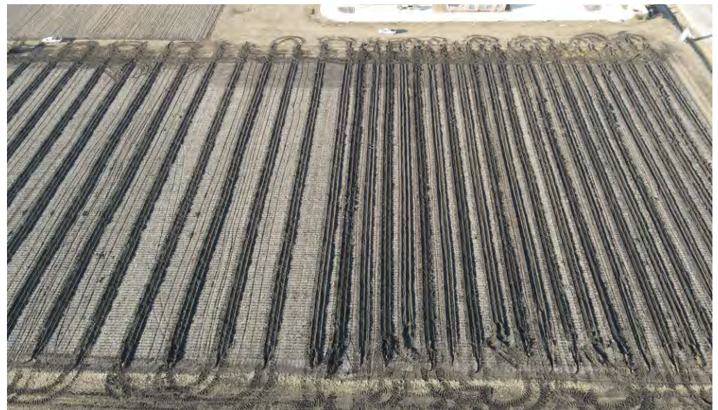
Figure 2. 15' and 30' Pattern Tile Installation
