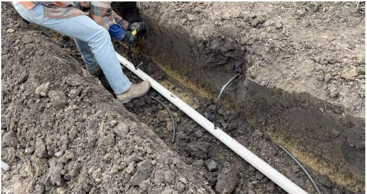
Figure 2. NETAFIM Sub-Surface Irrigation
