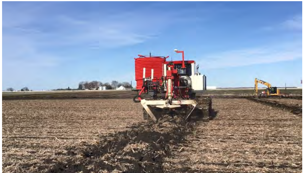
Figure 1. Tile Installation
