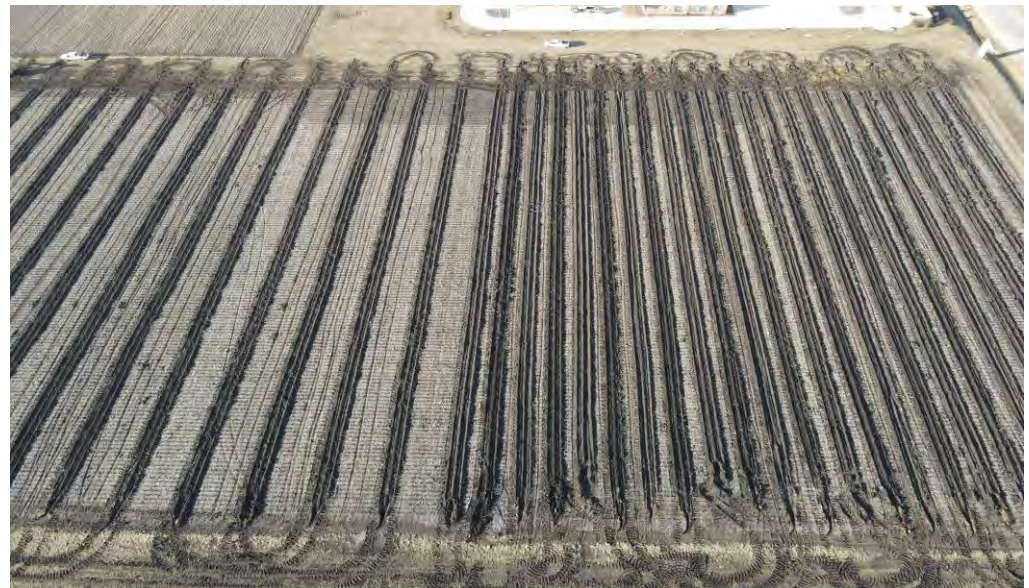
Figure 2. 15' and 30' Pattern Tile Installation
