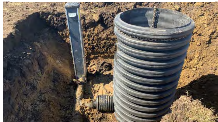
Figure 3. Gate Structures to Control Water Table
